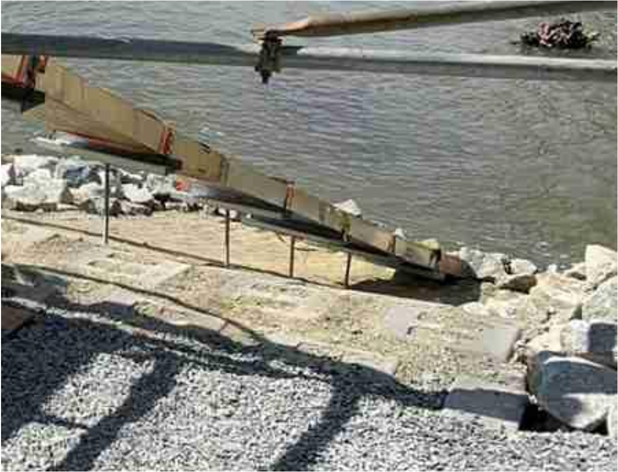
Figure 3.1-6: T-bar supports driven through ACBs, Octoraro Creek Eel Facility, 2024
