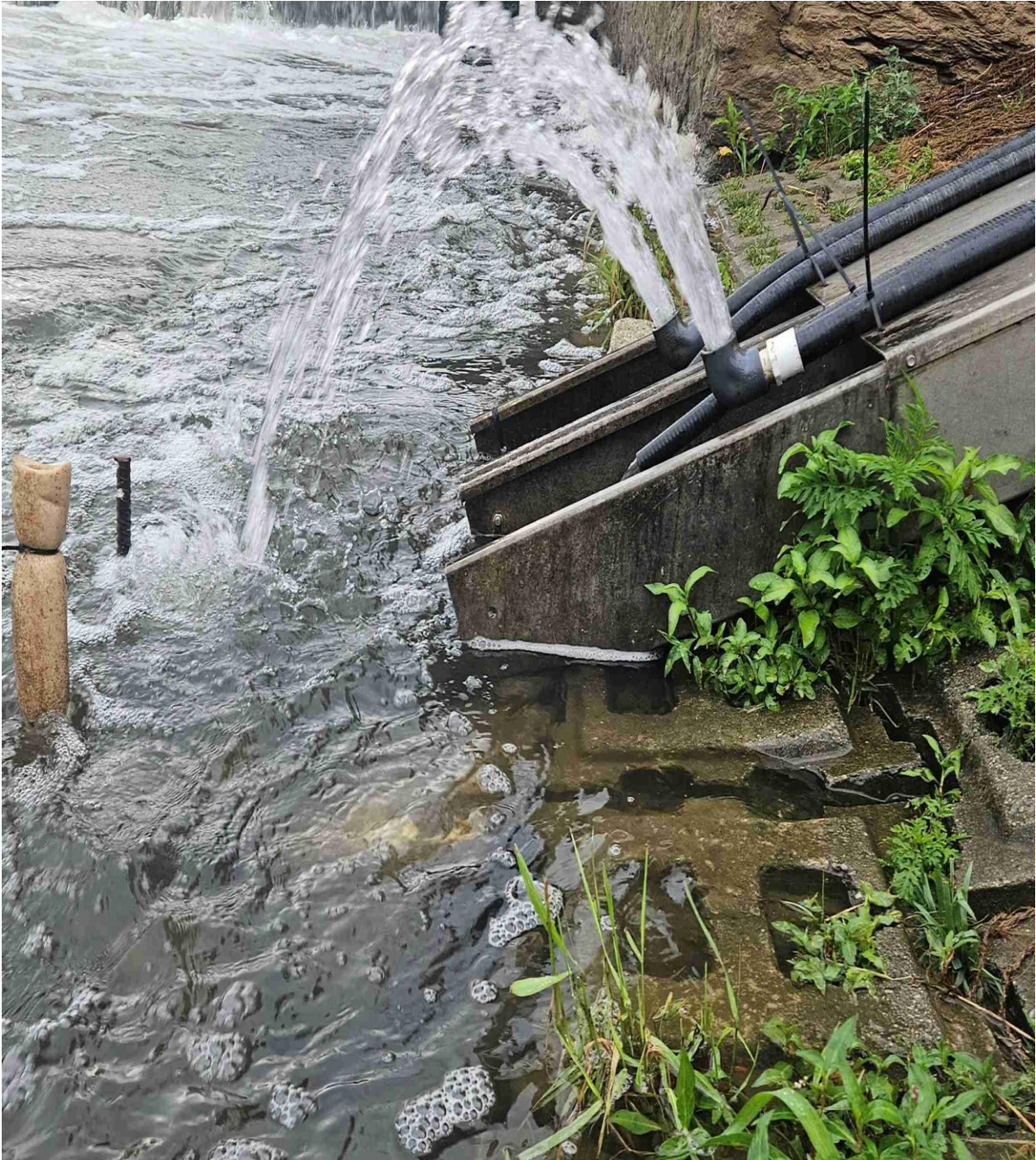
Figure 3.1-5: Ramp Entrance during 2024 Eel Collection Season at 191 cfs, Octoraro Creek Eel Facility, 2024
