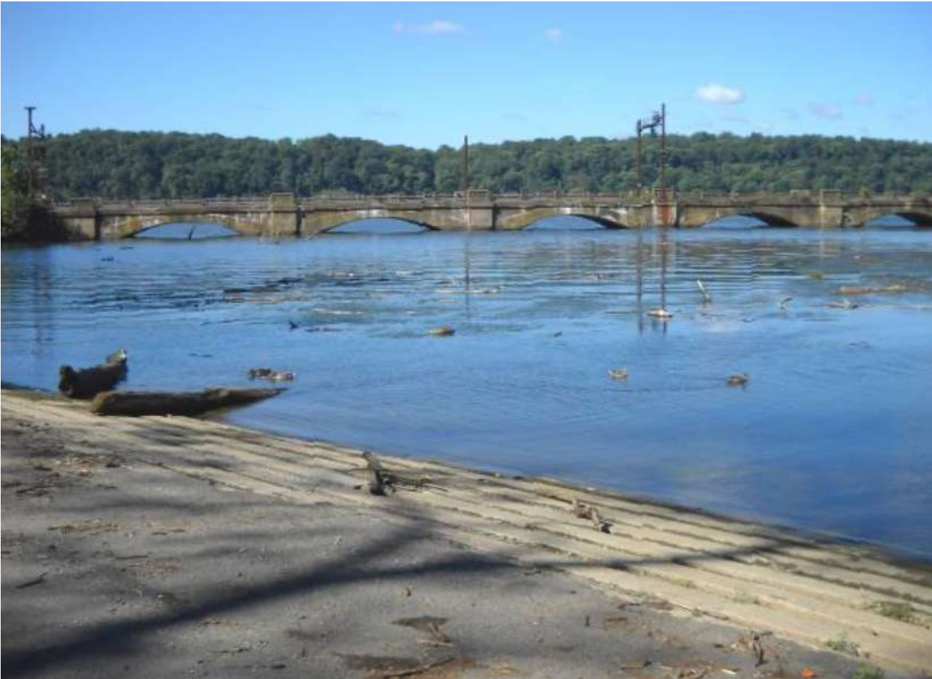
Figure 4.7-6: Conowingo Creek boat ramp (Site 1) Stocking Site, 2023
