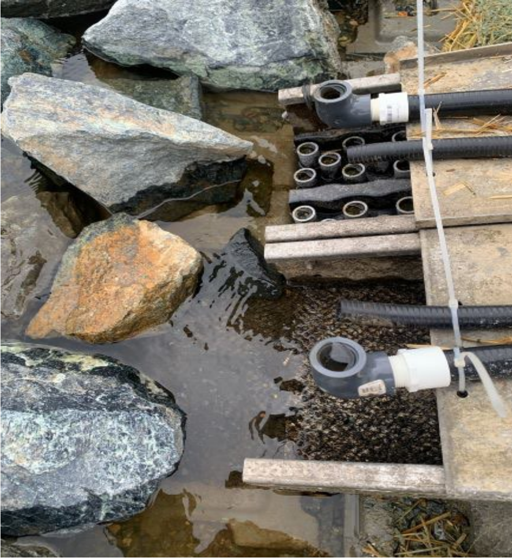
Figure 5.0-1: Ramp Entrance at ACBs (182 cfs ),Octoraro Creek Eel Facility, 2022
