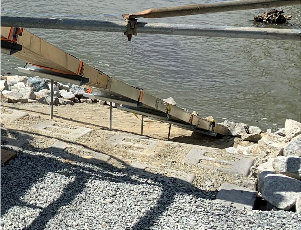
Figure 3.1-2: T-bar supports driven through ACBs, Octoraro Creek Eel Facility, 2022
