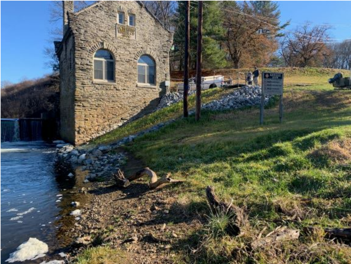
Figure 5.0-3: Bank Stabilization Project with Established Seed, Octoraro Creek Eel Facility, 2015-2022
