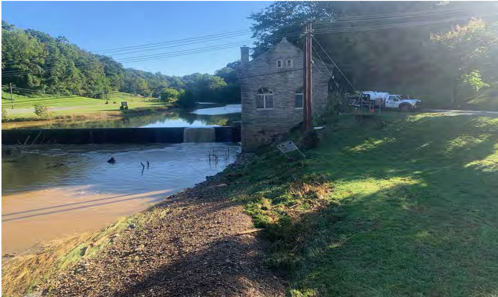
Figure 5.0-3 Damaged from High Creek Flows, Octoraro Creek Eel Facility, 2021
