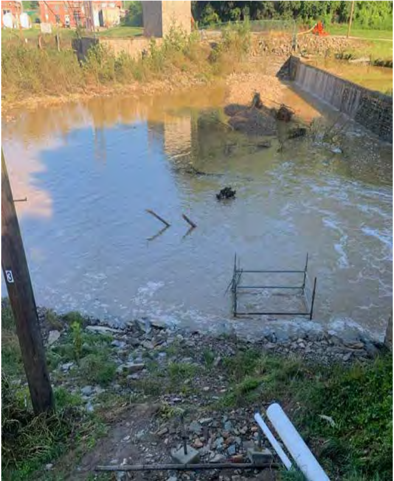
Figure 5.0-4 Changes in Tailrace After High Creek Flows, Octoraro Creek Eel Facility, 2021
