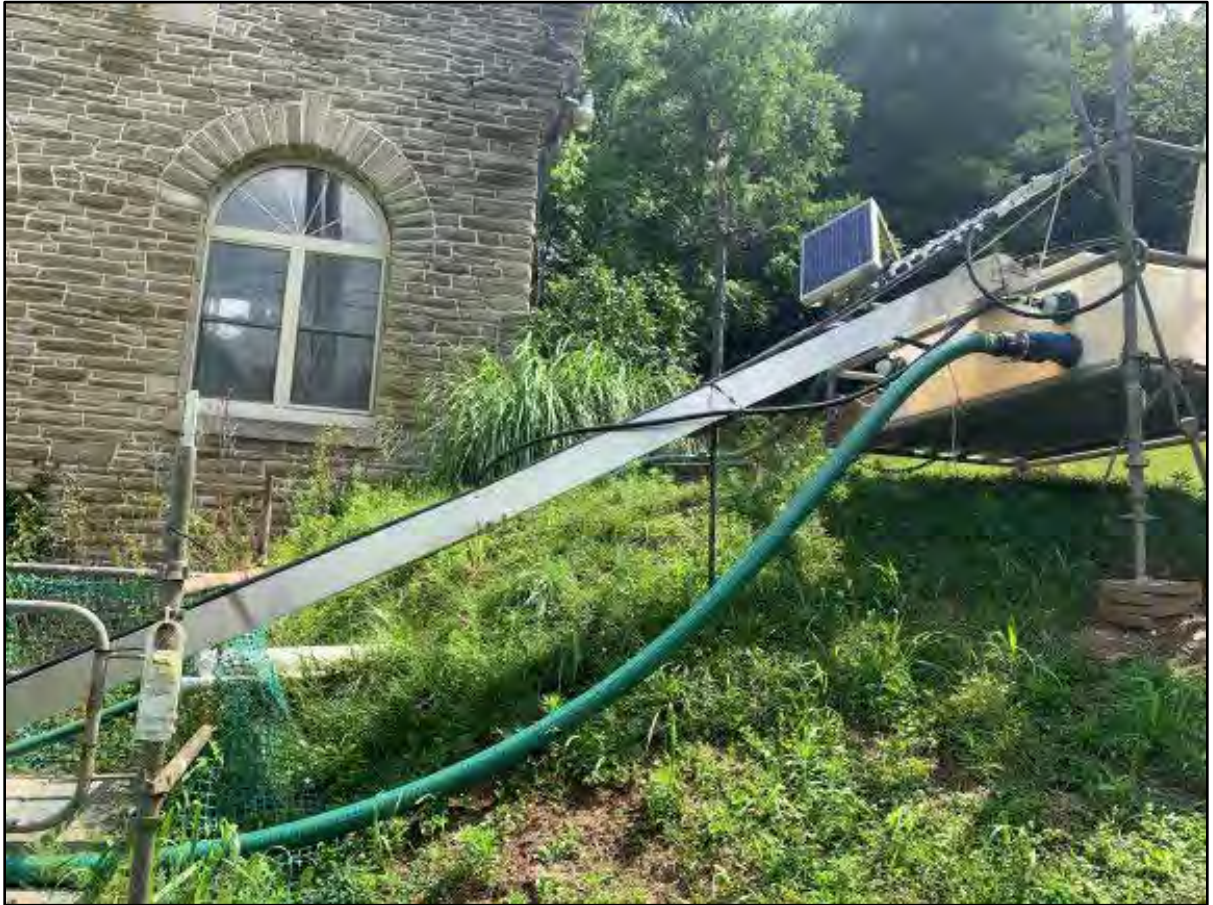
Figure 3.1-3: Braces and scaffolding supporting longer ramp, Octoraro Creek Eel Facility, 2021
