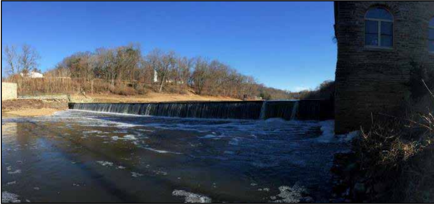
Figure 2.0-2: Location of the Juvenile Eel Collection Facility on South Shore (Left Bank) Of Octoraro Creek Downstream of Art Building
