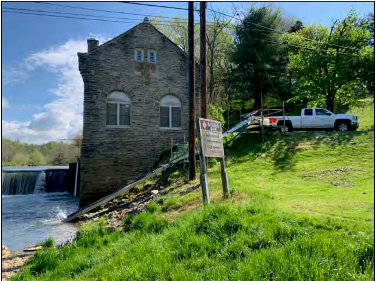
Figure 3.1-1: Scaffolding and Collection Tank on top of the hill, Octoraro Creek Eel Facility, 2021
