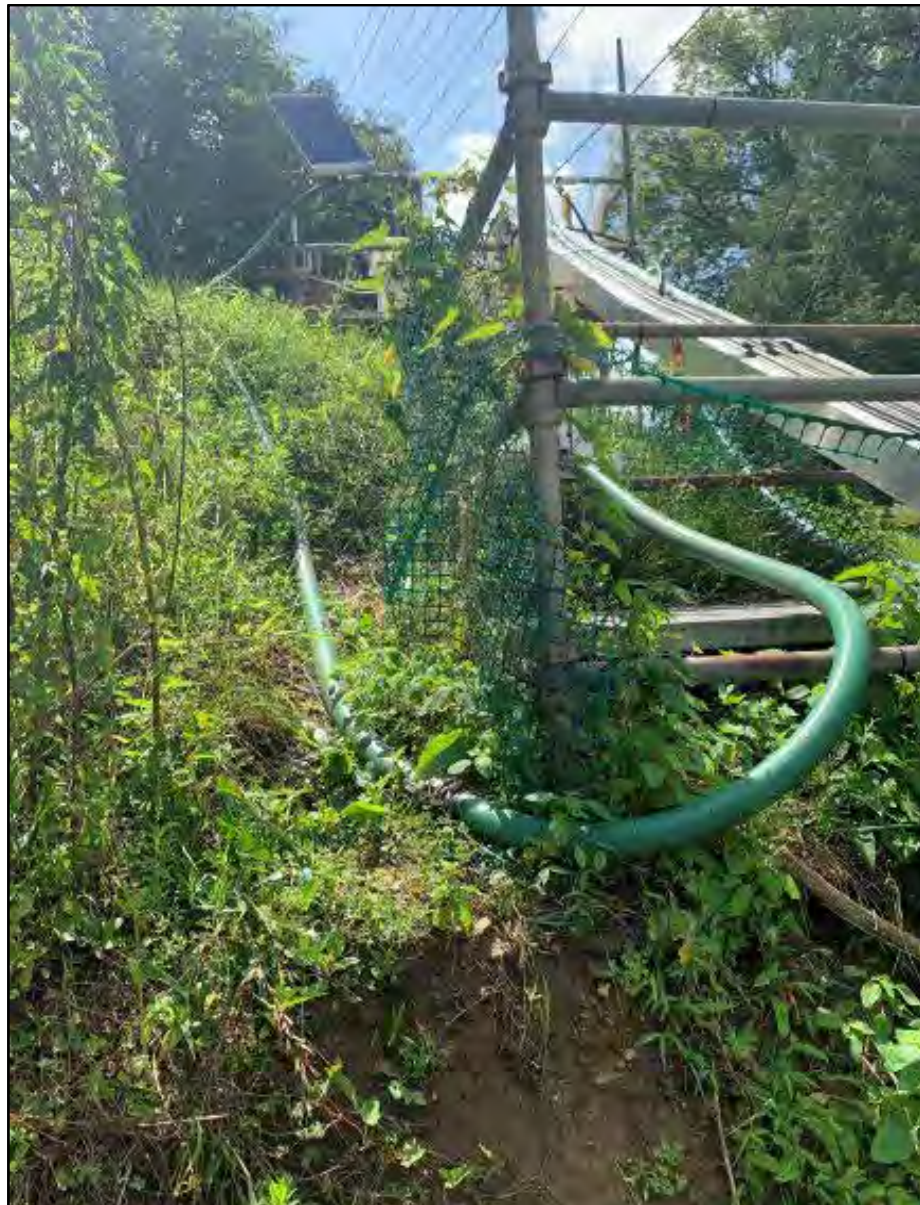
Figure 3.1-4: Additional length of hose for attraction flow, Octoraro Creek Eel Facility, 2021
