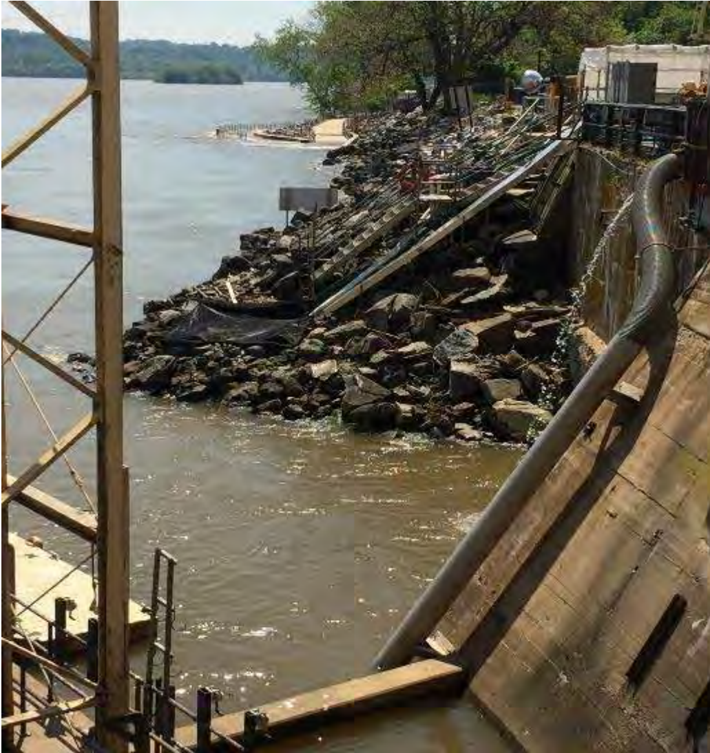
Figure 2.0-2: Location of the Conowingo West Eel Collection Facility Just Downstream of the West Fish Lift, Conowingo, MD, 2021
