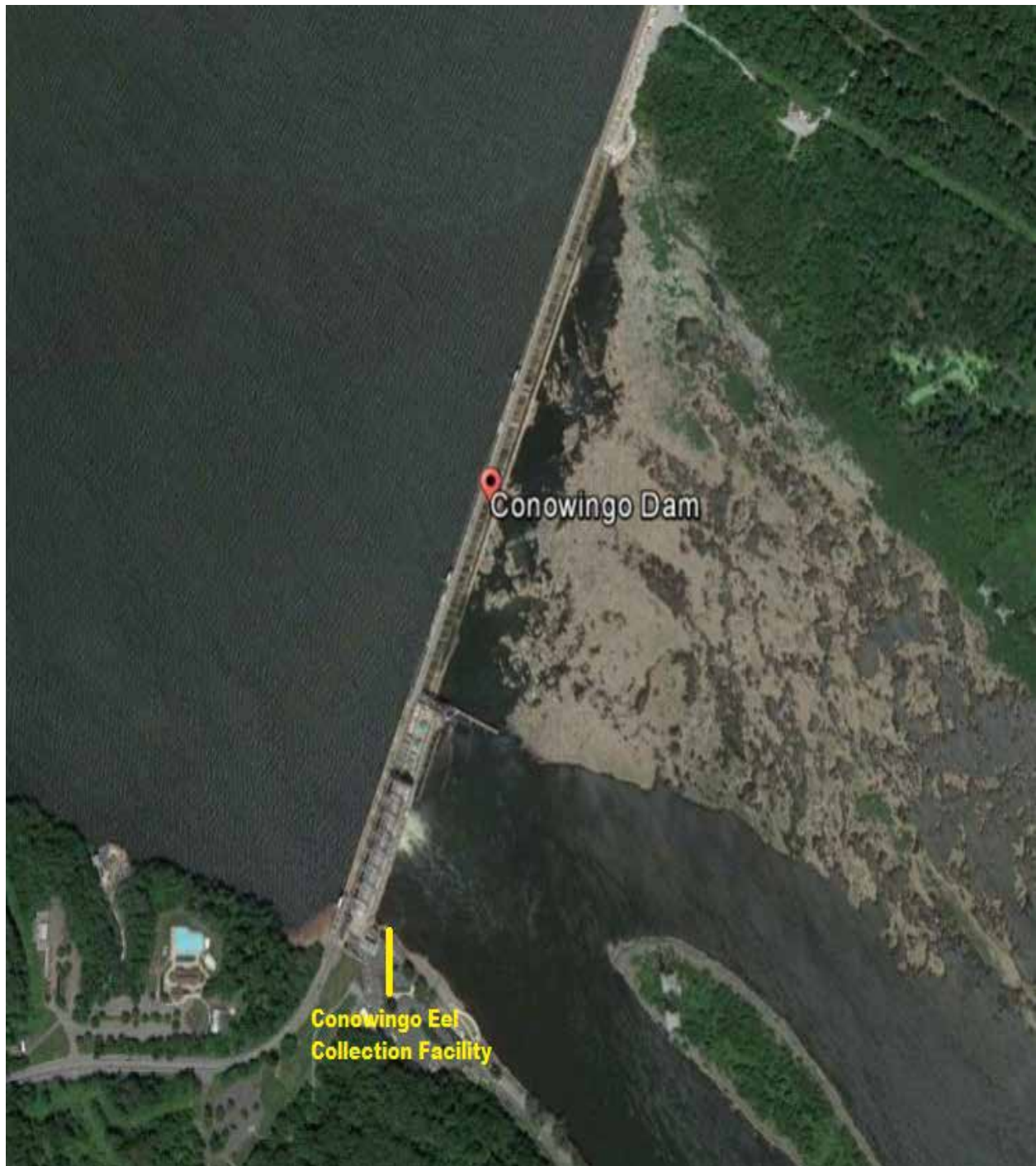
Figure 2.0-1: Location of the Conowingo West Eel Collection Facility at Conowingo Dam, 2021
