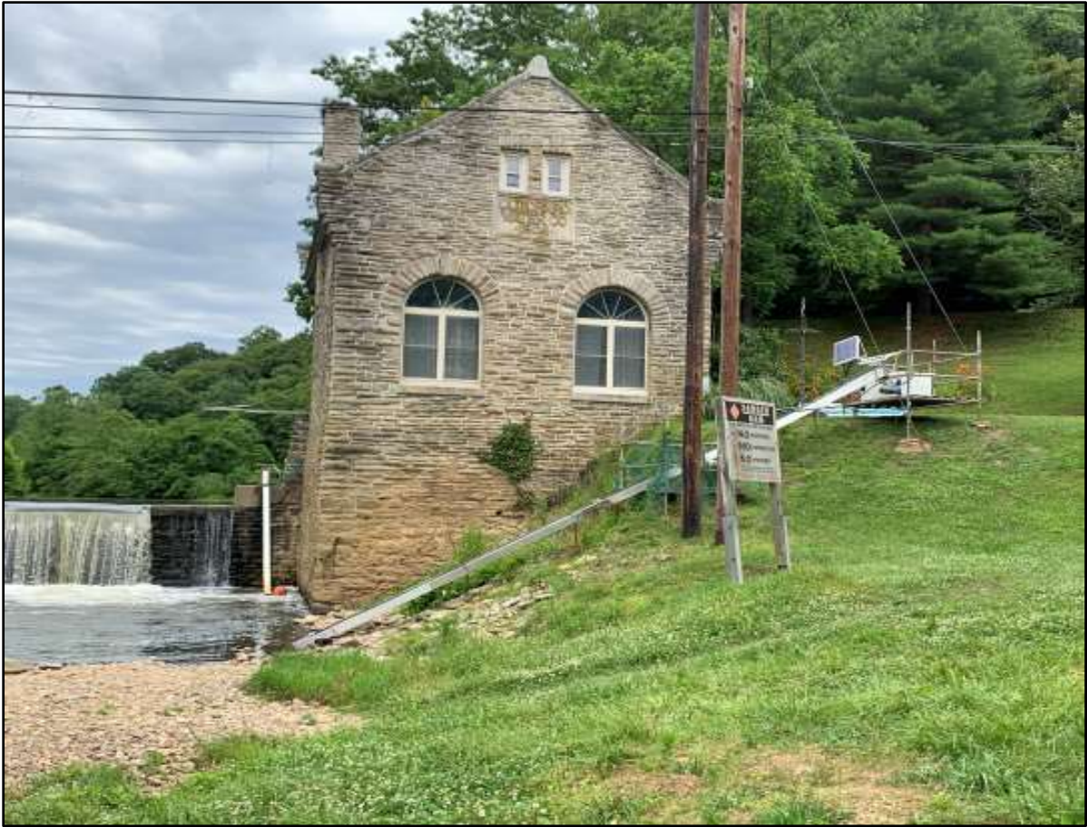
Figure 3.1-1: Scaffolding and Collection Tank on top of the hill, Octoraro Creek Eel Facility, 2020
