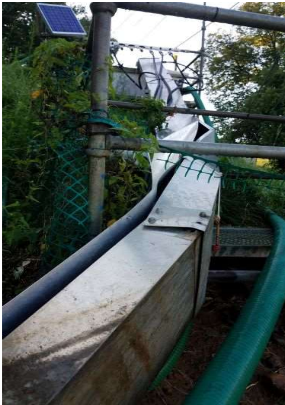
Figure 5.0-3 Damaged from High Creek Flows, Octoraro Creek Eel Facility, 2020
