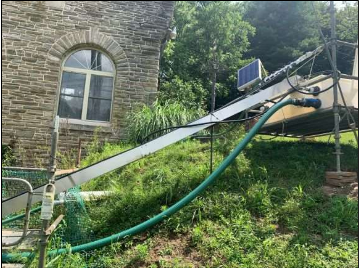
Figure 3.1-3: Braces and scaffolding supporting longer ramp, Octoraro Creek Eel Facility, 2020
