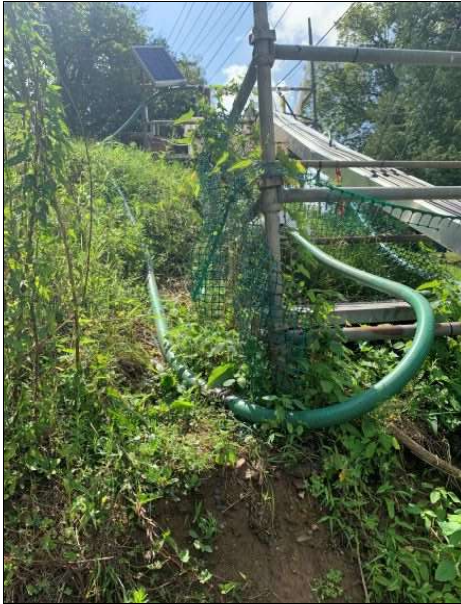
Figure 3.1-4: Additional length of hose for attraction flow, Octoraro Creek Eel Facility, 2020
