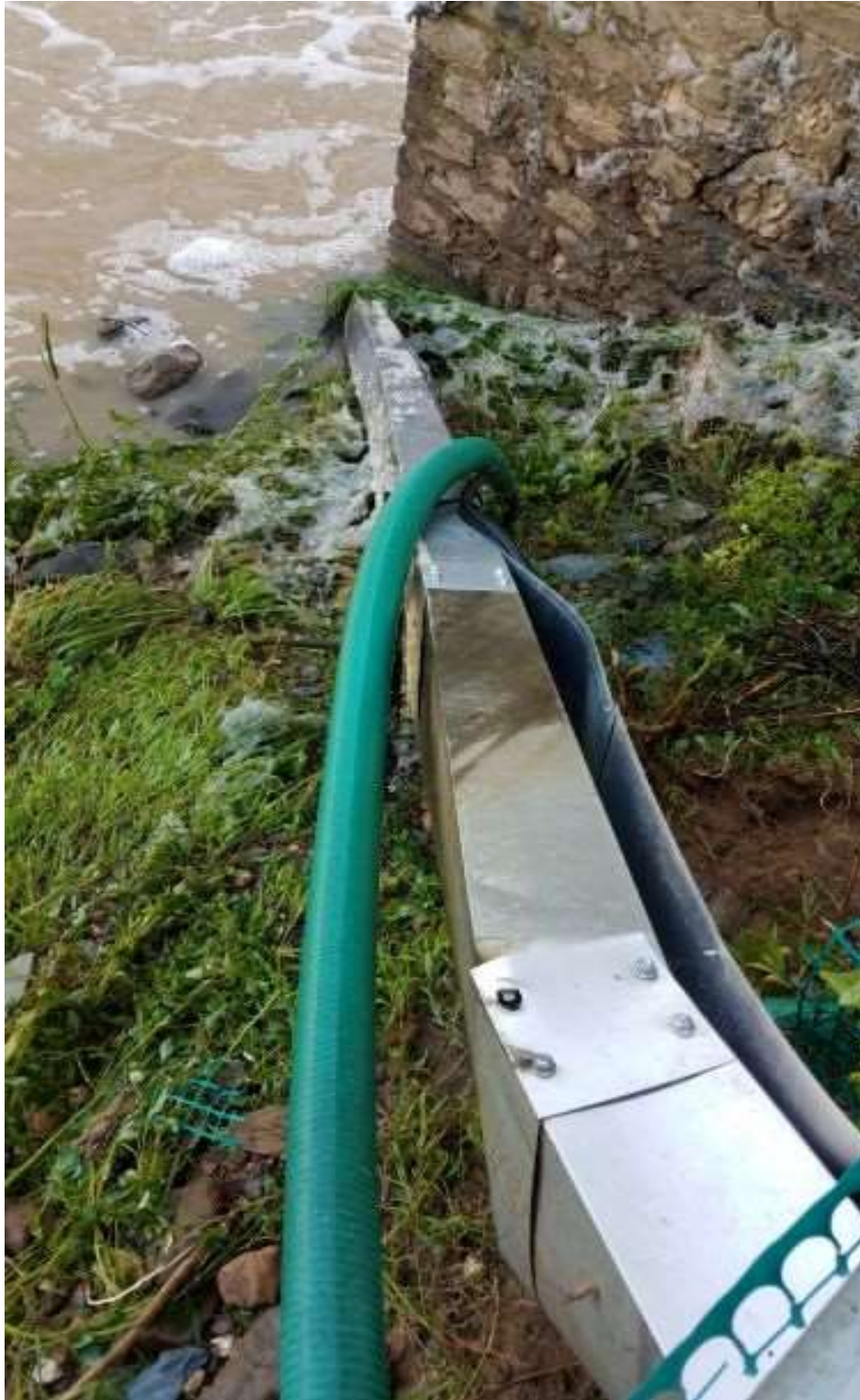
Figure 5.0-4 Damaged from High Creek Flows, Octoraro Creek Eel Facility, 2020
