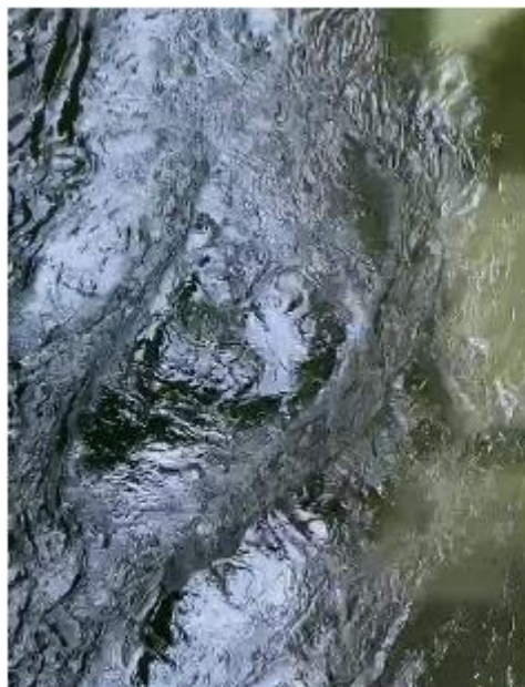
Photo 3: Upwelling along spillway lift channel wall downstream of turn with matrix settings
