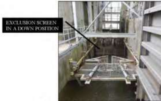
Figure 1 - Exclusion screen in down position during fishing mode
