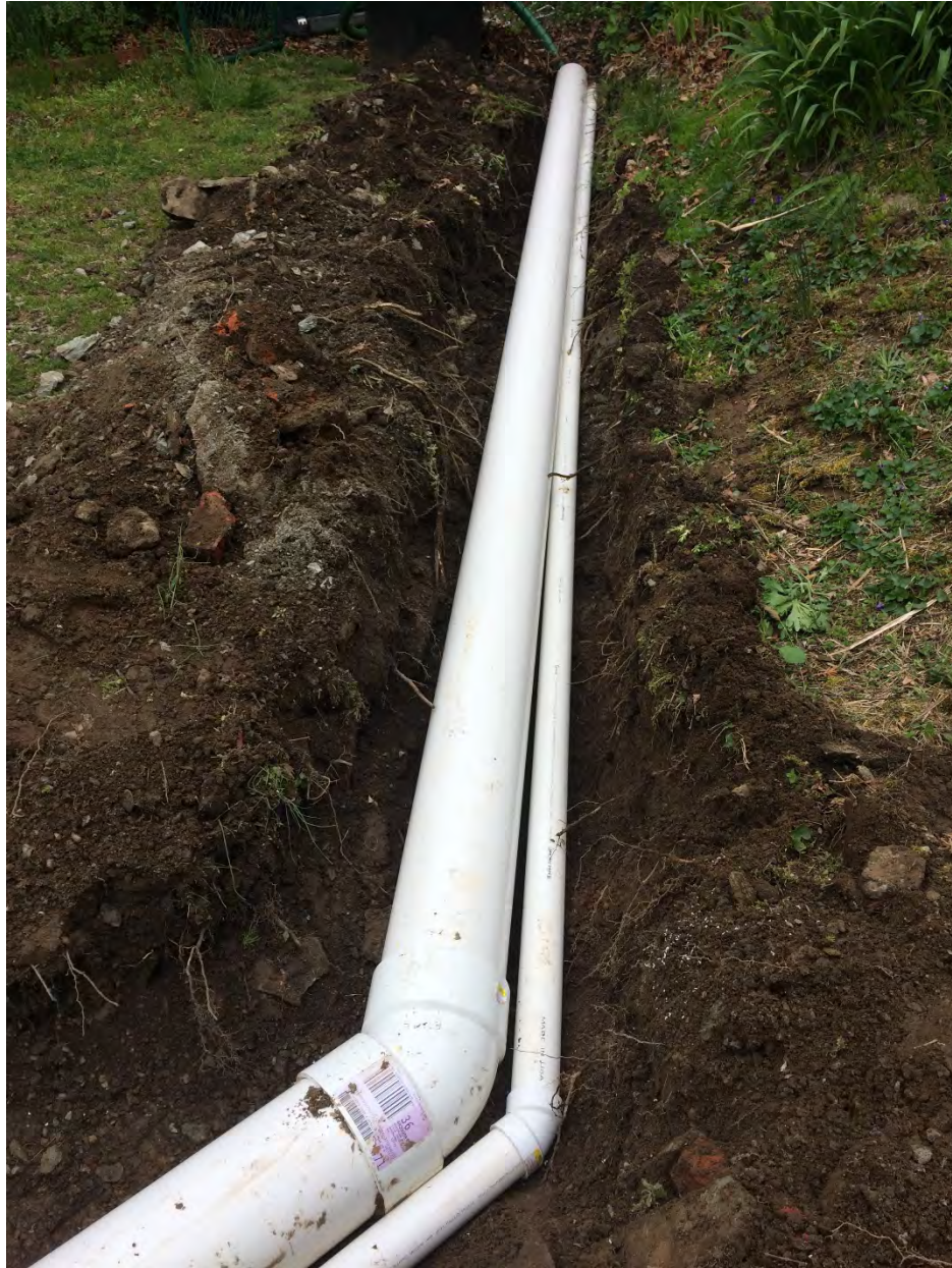
Figure 3.1-3: Larger Water Line Placed Underground, Octoraro Creek Eel Facility, 2019
