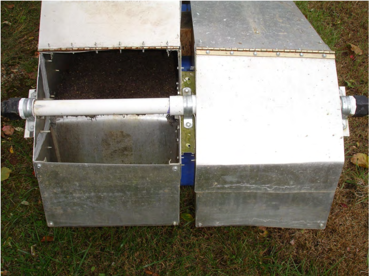
Figure 3.1-1: Hinged Cover over Spray Bar to Decrease Light inside the Eel Ramp, Octoraro Creek Eel Facility, 2019
