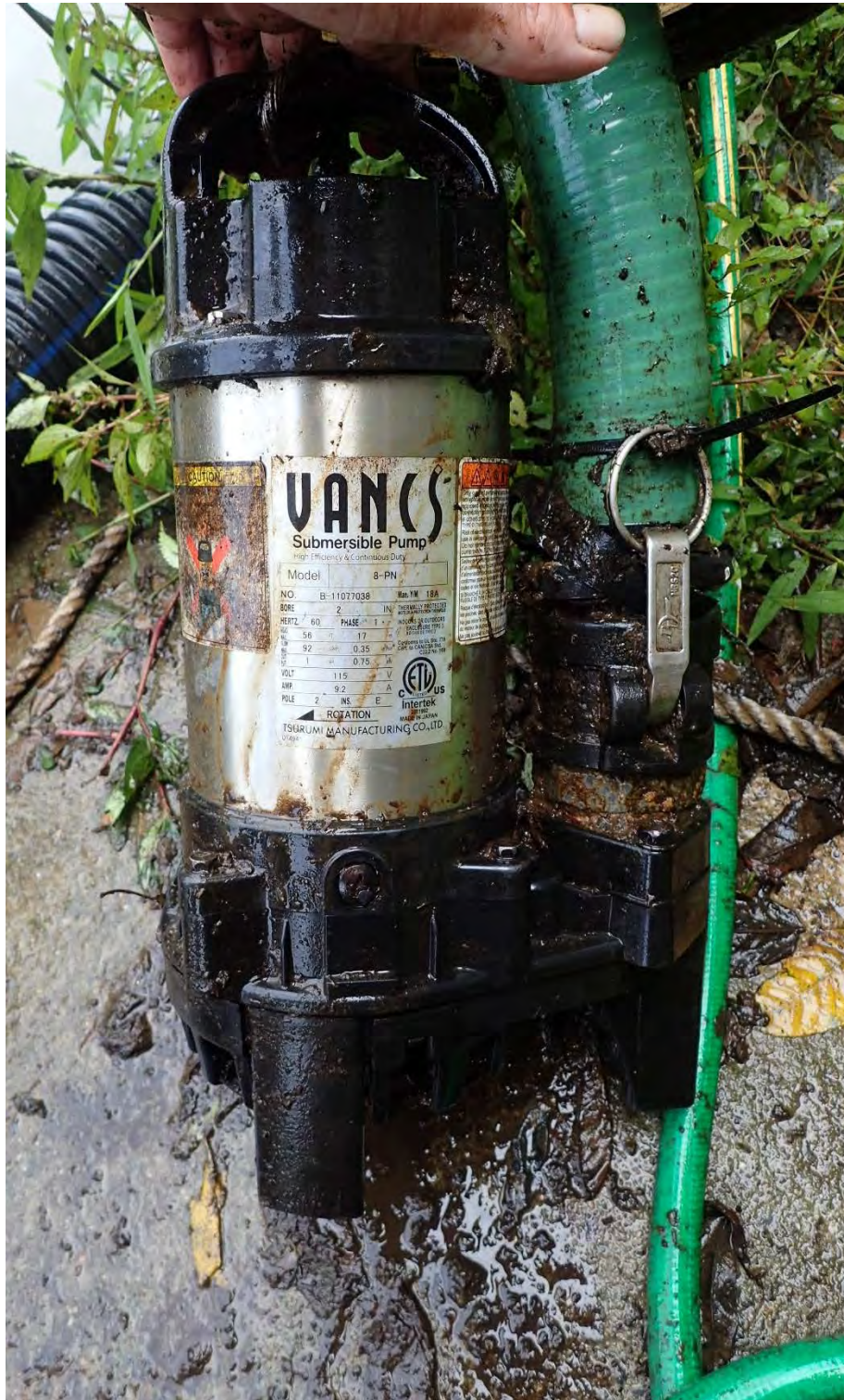
Figure 3.1-2: Submersible Pump for Attraction Flow, Octoraro Creek Eel Facility, 2019
