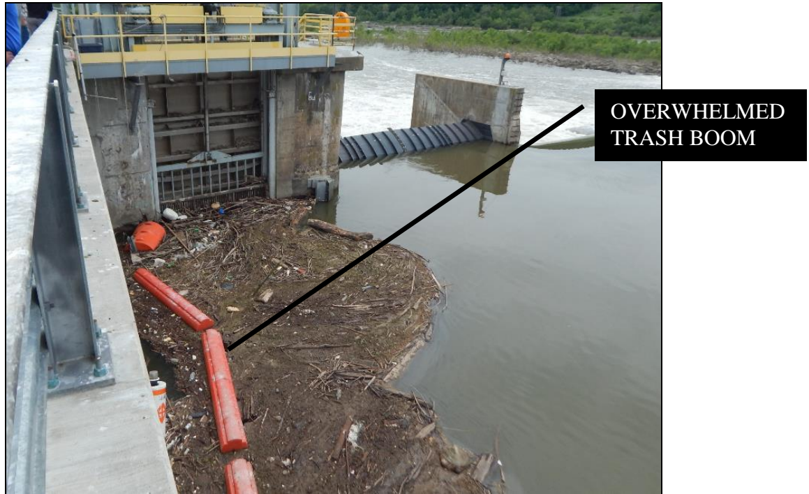
Figure 3 - Debris accumulation in the vicinity of the exit through trash rack
