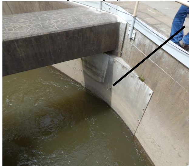
BOLT PROTRUDING INTO THE ZONE OF PASSGE
