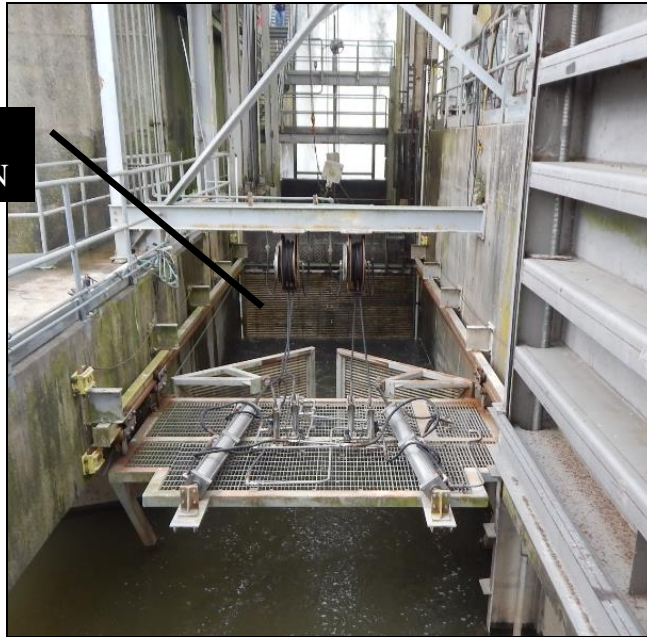
Figure 1 - Exclusion screen in down position during fishing mode
