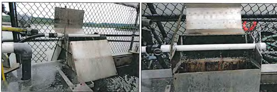
Figure 2 - Eel pass attraction flow entering the eel ramp vertically
