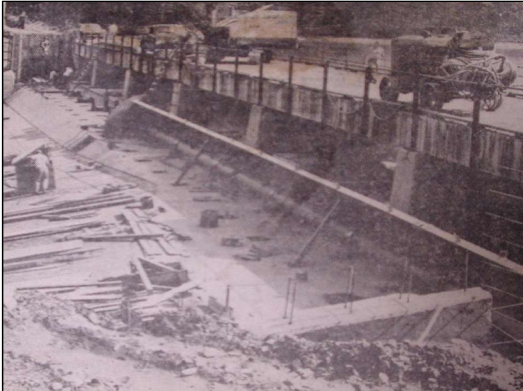
1955 – installation of bascule gates at Lake Williams to increase the lake level by 4 feet
