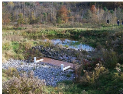
AMD water flows into the oxic limestone drain (OLD) and dissolves limestone, which increases the alkalinity and pH of the water.
