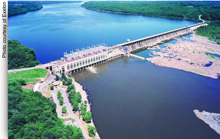
Looking north at the Conowingo dam with the pond in the upper portion.
