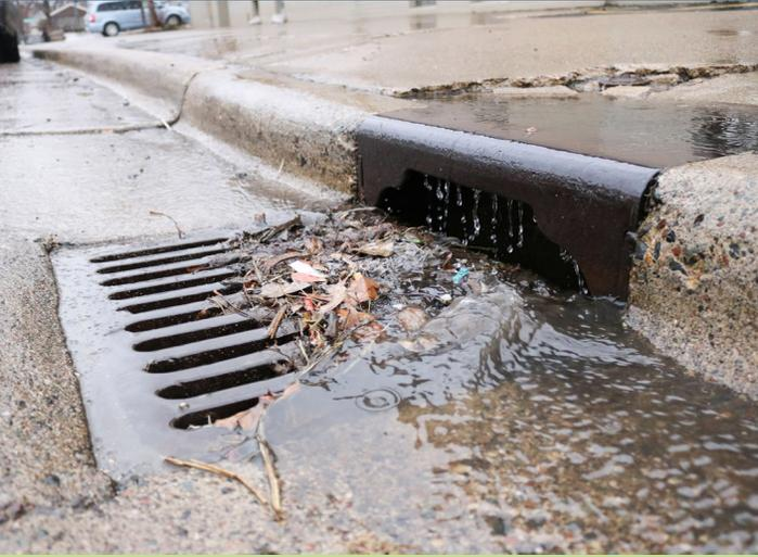
Rain that falls on impervious surfaces — roofs, parking areas, and roads — flows off these surfaces until it finds a storm drain or a place to soak into the ground. Along the way, the runoff picks up pollutants like trash, oil, pesticides, fertilizers, and sediment.
