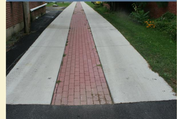
Limekiln Alley in Wrightsville Borough is York County, PA's first green alley. It allows rain water to infiltrate through pervious brick pavers, beneath which there is a drain field with stone and a perforated pipe.
